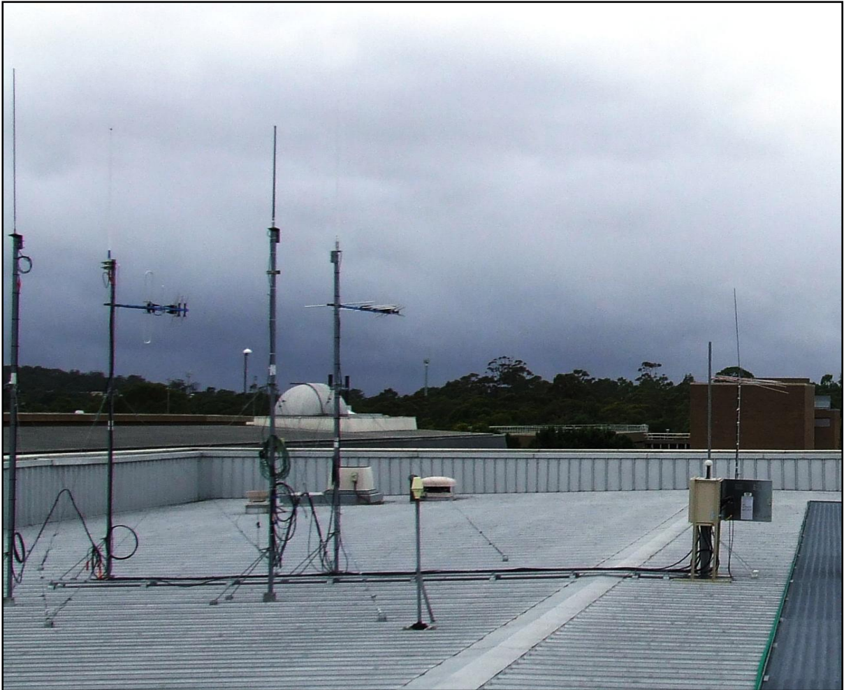
Figure 1: Antennas on the Rooftop of BG Building as a Base Station – One of these antennas is the scanner antenna that connected to Field Strength Analyser
